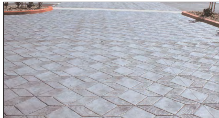
Concrete parking delivers versatility: Concrete surfaces can be placed with an array of textures, shapes, patterns and colors.
