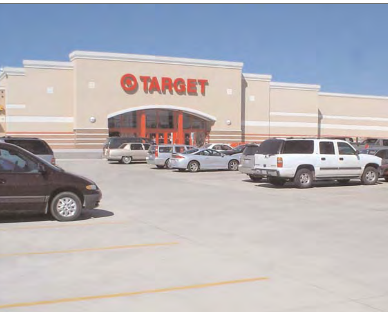
Concrete parking delivers curb appeal: Bright, white concrete enhances any property. Plus, increased reflectivity can lower cooling and lighting costs.
