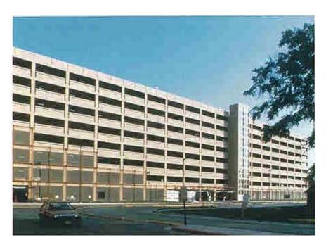
had the lowest life cycle cost. Another important factor that influenced the decision to use a cast-in-place beam and slab system was the clean, relatively flat underside of the structure. This provided enhanced lighting. The improved lighting addressed the Owner's concern for safety in the 24-hour a day garage.
